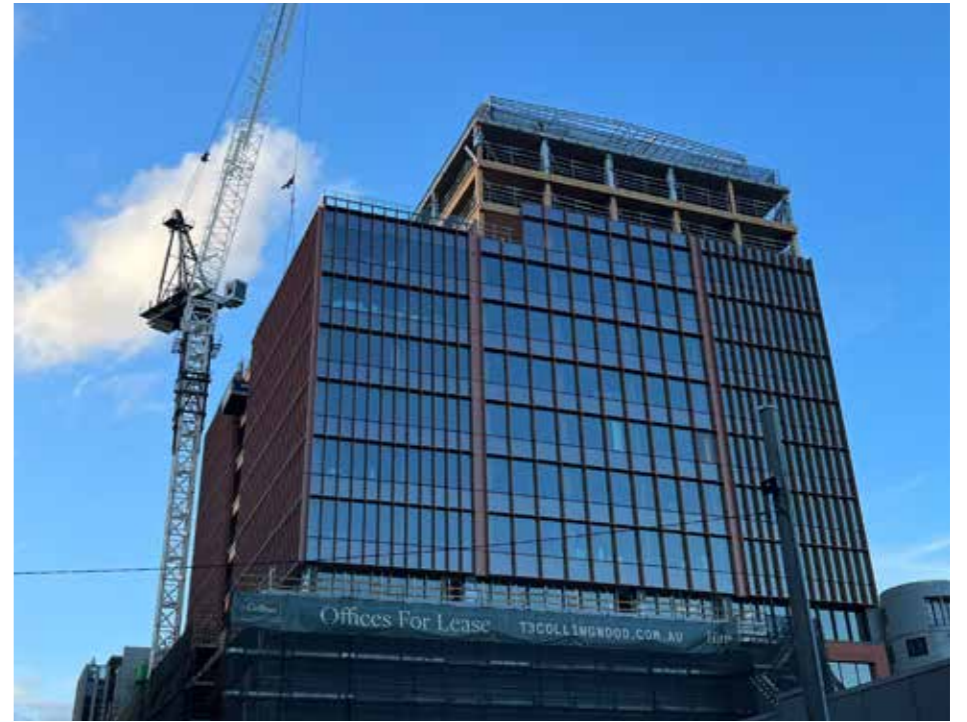
Rising up & topping out
